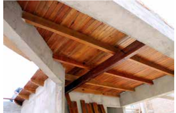
This is the first ceiling to be put in place in the house. We are using wood beadboard to reflect the beautiful Spanish colonial style of Honduras' origins.
