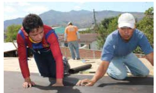
Micah 11th grader Moises helps to lay the asphalt cover on the wooden ceiling above the new bedrooms.
